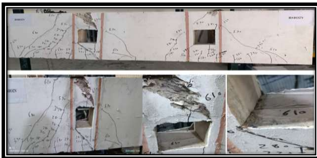
Figure (21): Crack patterns and failure mode for specimen (BSIO2V)
