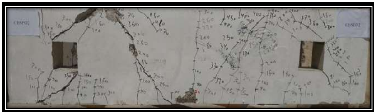
Figure (13): Crack patterns and failure mode for specimen (CBSEO2)
