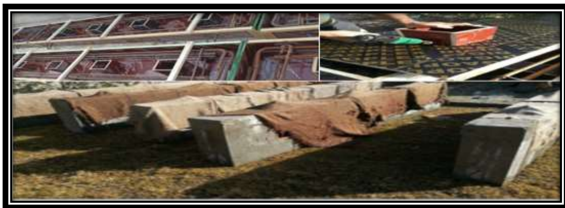
Figure (8): Casting and Curing Process
